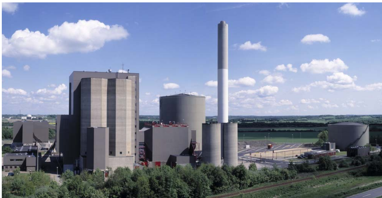
CHP plant in Herring, Denmark (source: Elsam)
