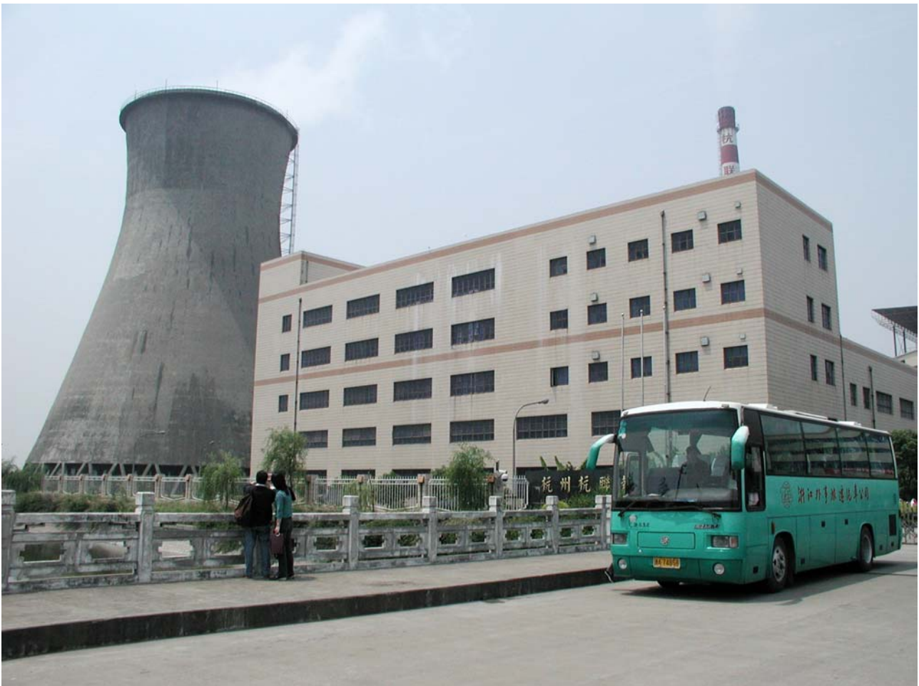
CHP plant in Hangzhou, China
